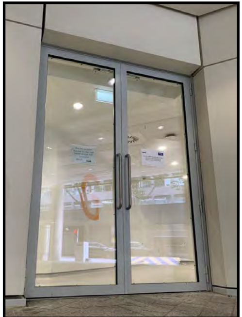
ABOVE: (left) Premier's tested LPS1175 SR3 (C5) security and FB4 Ballistic Glazed system (Right) Premier's tested LPS1175 SR4 (D10) security and FB4 Ballistic Glazed system
